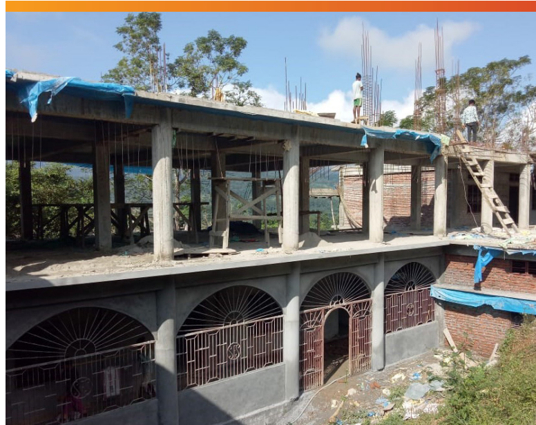
Above: Ongoing school building construction
