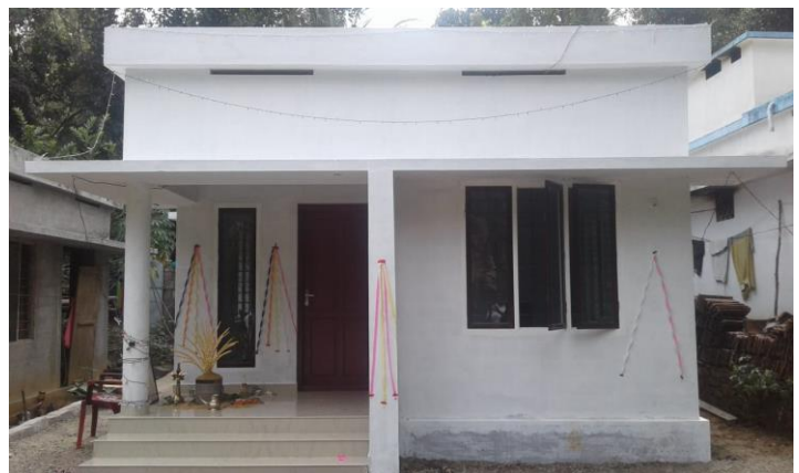
Above: new House
