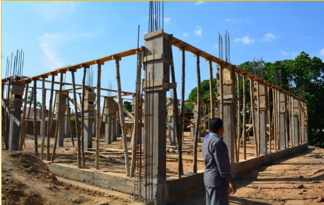
Above: Start of construction of the new School Building
