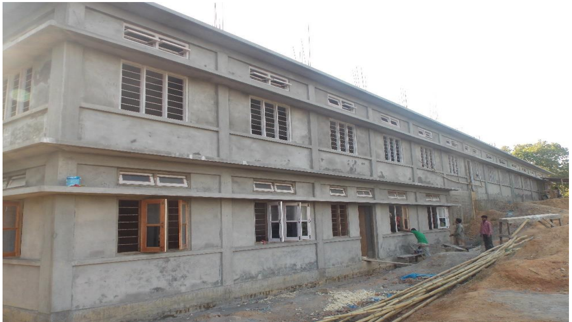
School building shortly before completion
