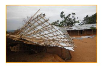
A school building made of a bamboo and palm-leaf roof (see pictures below) has been completely destroyed after the storm over Easter 2015. The village urgently needed a school with solid walls, a stable roof and the necessary infrastructure to meet future needs.
