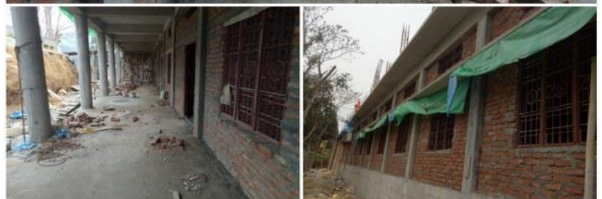
Right: Status of the construction work end of 2019
